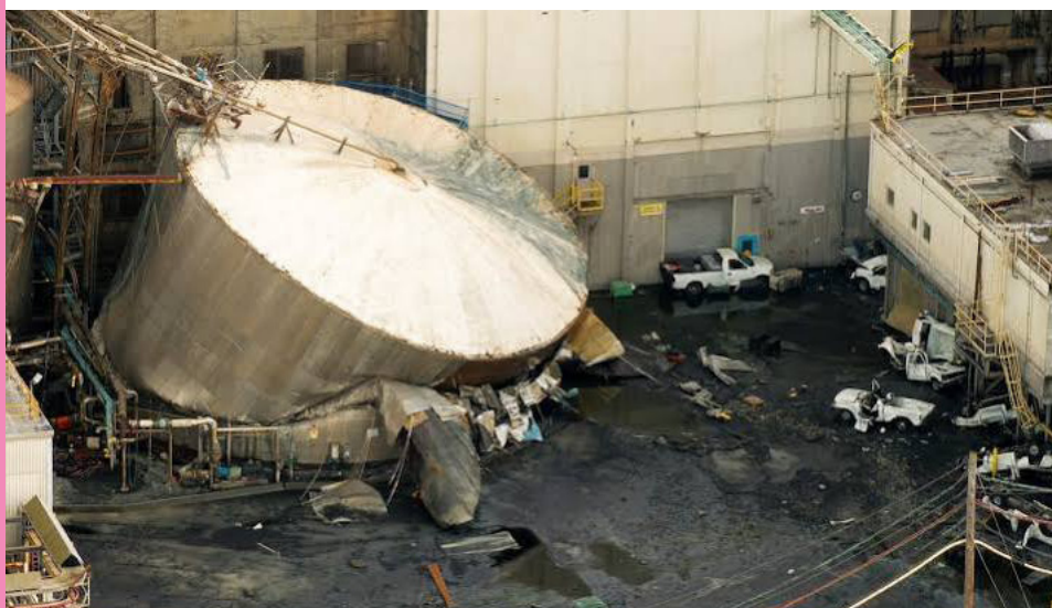
Tank collapse at Longview, Washington, killed 11 people.
