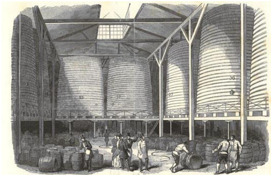
The vast size of London's beer vats is illustrated by this sketch of the Barclay and Perrin's brewery in 1847, after construction standards were changed from wood.
